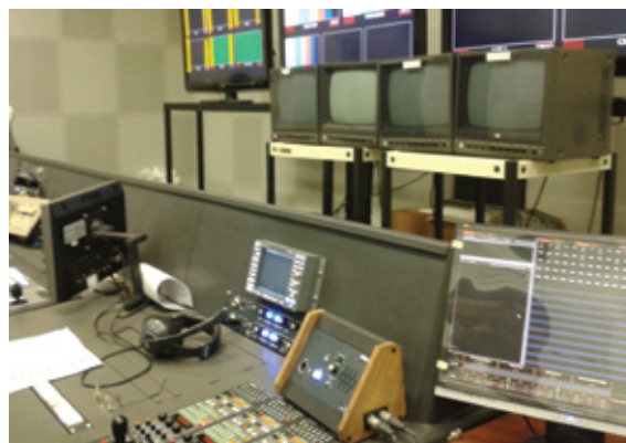
Figure 6e: Transformation of audio-visual equipment in the studio complex to hi-definition status in 2009
